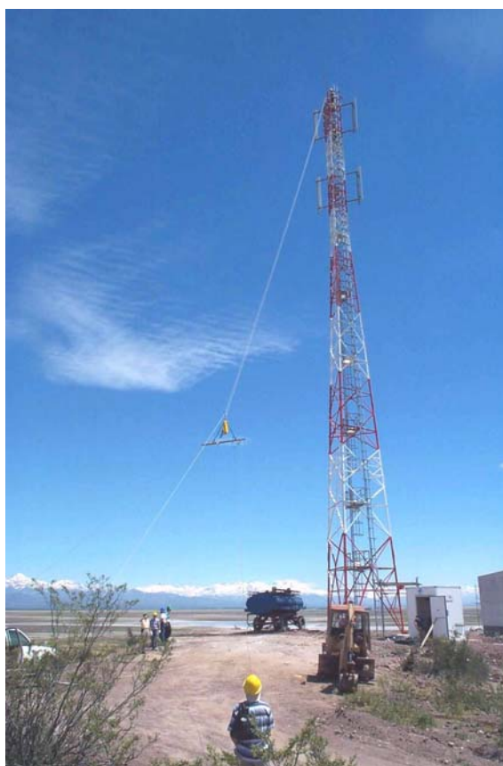
Figure 3.1.6: Installation of WLAN panel antennas on the 41 metre tower at Los Leones
