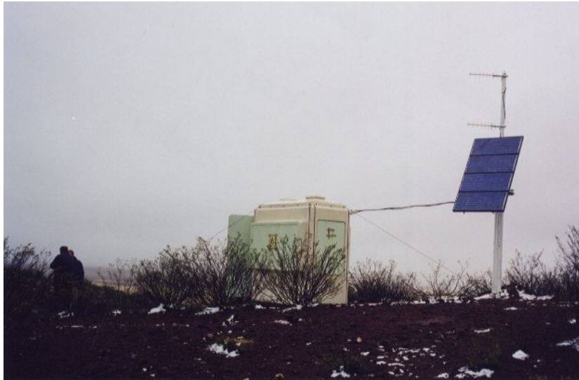
Figure 3.4.5 : Los Leones base-station controller shelter (Dec 1999 - May 2001)
